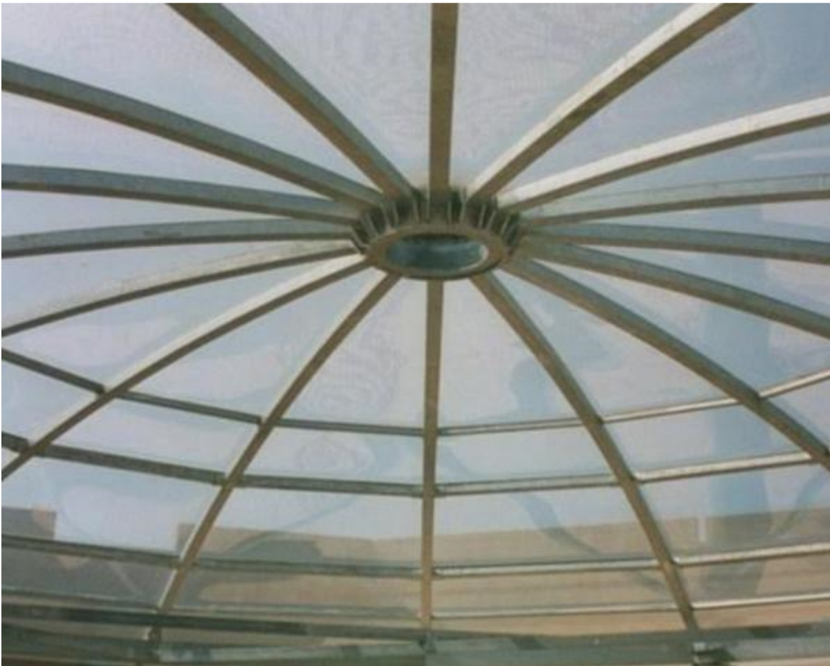
Solid plates MACROLUX® Example of transparent roof made of slabs MACROLUX® Solid
