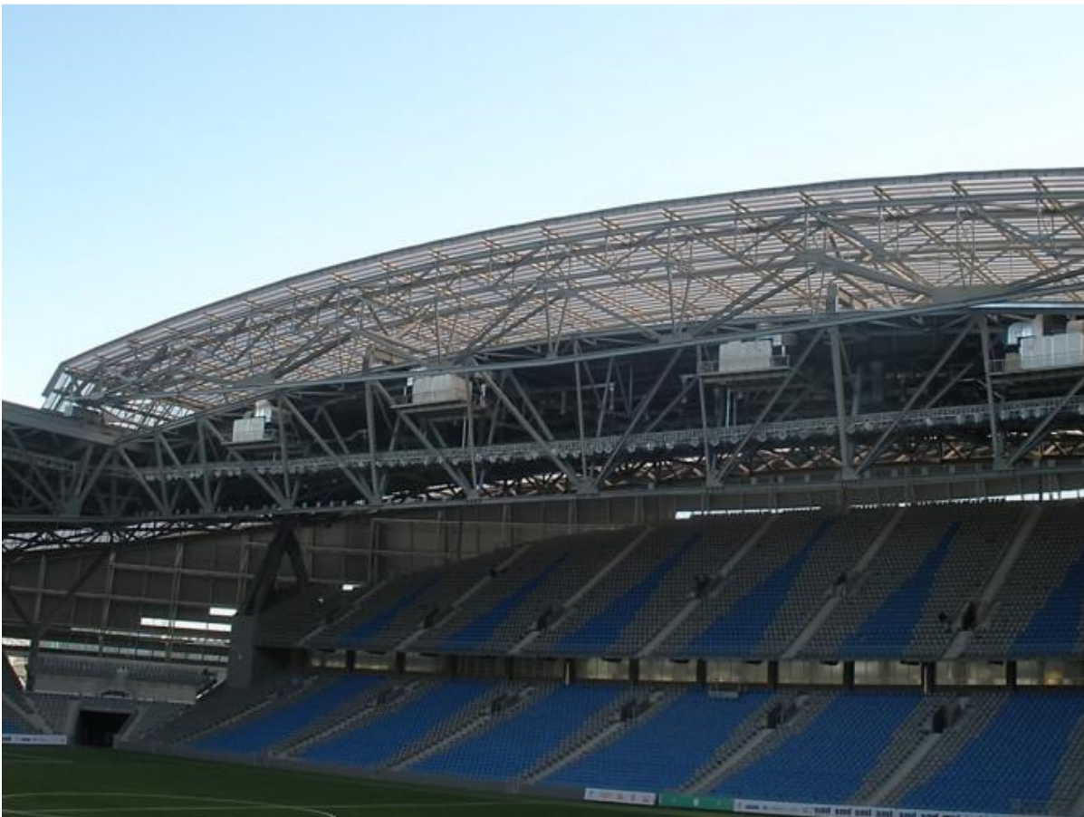
Astana Stadium Coverage Stadium, Astana (KZ) - 2007 - exemplary embodiment with the use of plates MACROLUX® Multiwall.
